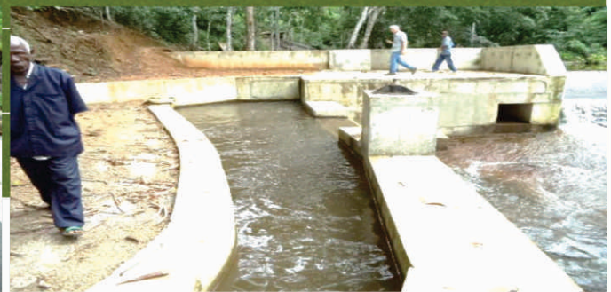
Spillway & In-take Complete
