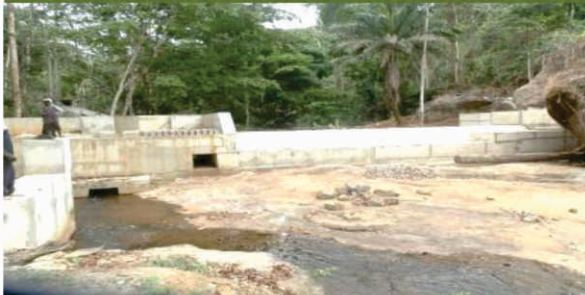
Spillway & In-take Complete
