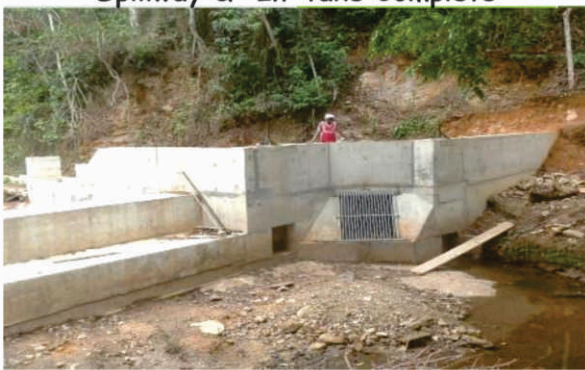
Spillway & In-take Complete
