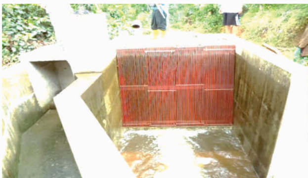
Spillway & In-take Complete
