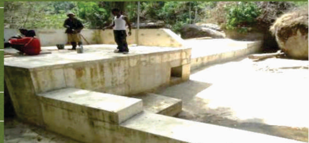
Spillway & In-take Complete
